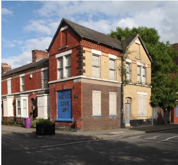
Derelict properties at the junction of Granby Street and Cairns Street
